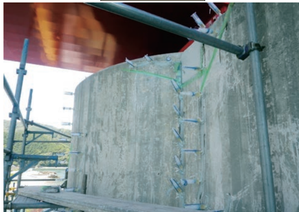
ひび割れ補修
